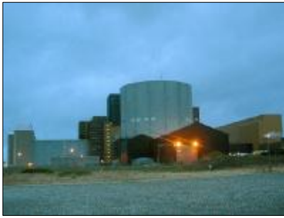
The power station is located in Anglesey
