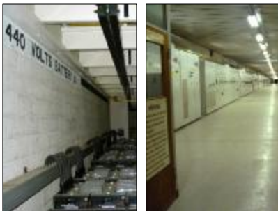
Plant rooms required careful dust control
