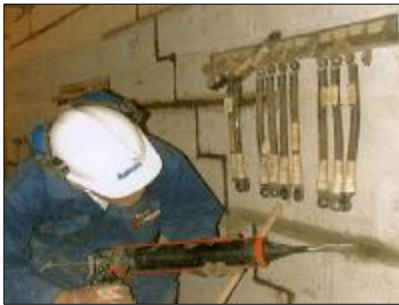
Gun applying the bedding mortar
