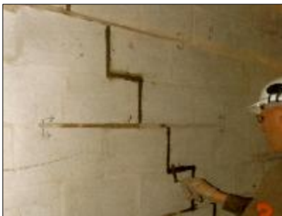
Pointing up the repair
