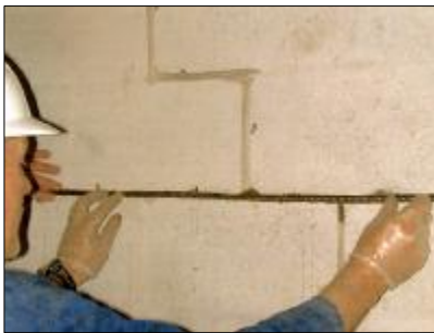
Laying in the stainless steel Helibar
