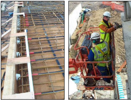
Live end anchors (L) Rebate filling (R)
