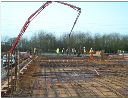
PT floor slab during casting
