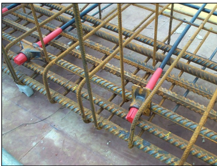
Dead end anchors prior to casting
