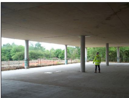
PT provides flat soffits and large spans
