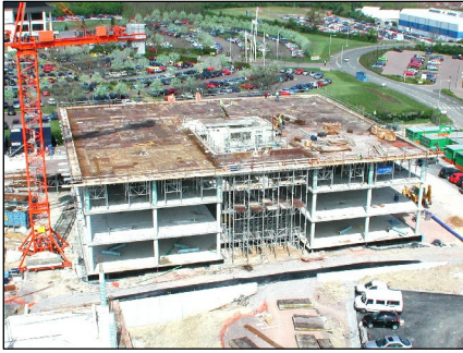
The first building at topping out stage
