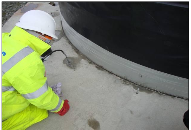
Photo Top : Injection packers in position
