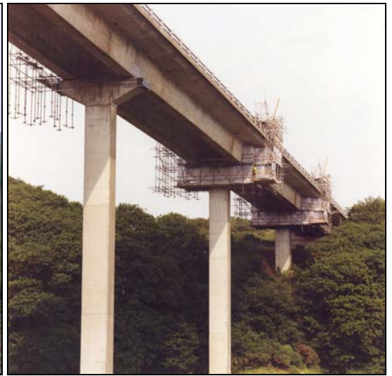
Suspended scaffolding provided access to
