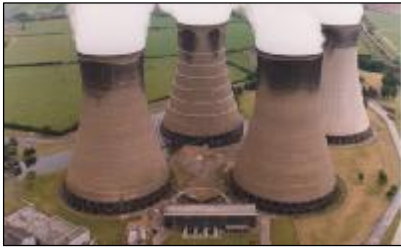
Cooling tower C1 (middle back)
