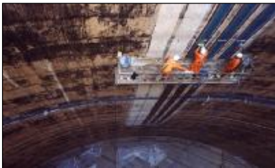
Work inside the tower was from cradles
