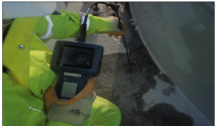
Balvac operatives undertaking specialist repairs, breakout, drilling, inspection, injection and repair
