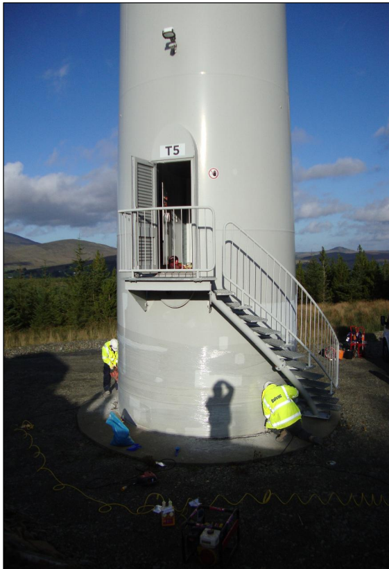
Balvac operatives undertaking specialist repairs, breakout, drilling, inspection, injection and repair
