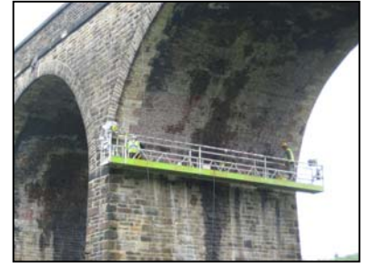
Brickwork repairs from cradle access
