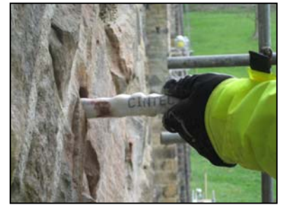
Installation of Cintec Anchors
