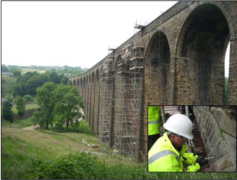
General view of Thornton Viaduct (inset - grouting works)
