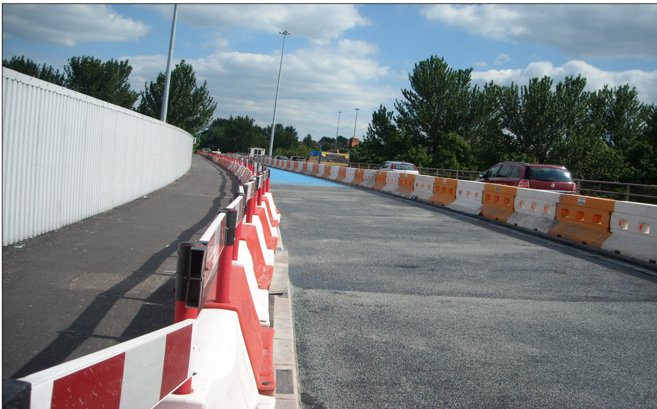
Image of the Runcorn Approach Viaduct nearing completion.
