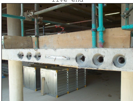
Anchorage pockets ready for filling
