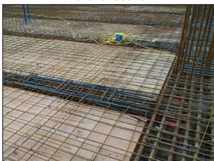
Dead end anchorage detail
