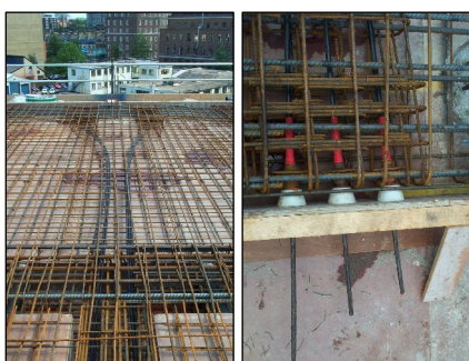
Unbonded tendons splay at the live end
