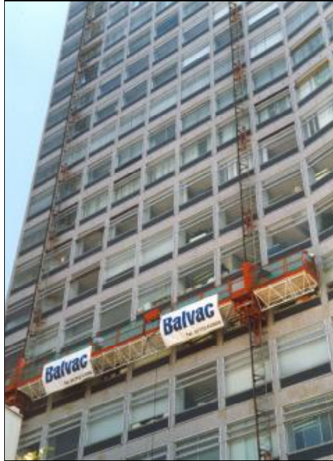
Mast climber and cradle access was used for all elevations
