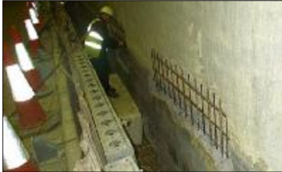
A deep trench was needed for access
