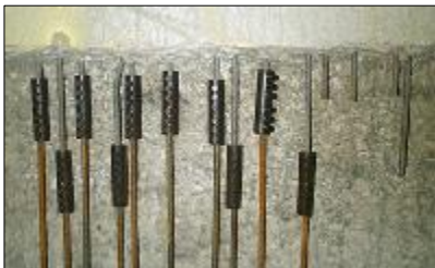
Nearly 5,000 rebar couplers used
