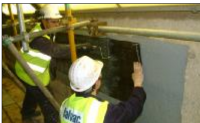
Carbon fibre composite strengthening
