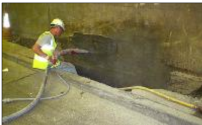
Spray concrete repair underway
