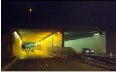
North portal during night-time possession
