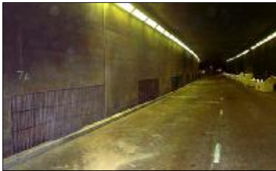
Hit and miss bays on the side wall
