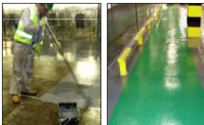
The floor was re-coated after repair
