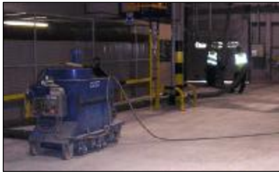
Grit blasting the floor slabs
