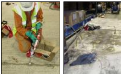
Cracks and voids resin injected
