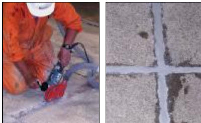
Joints repaired and sealed
