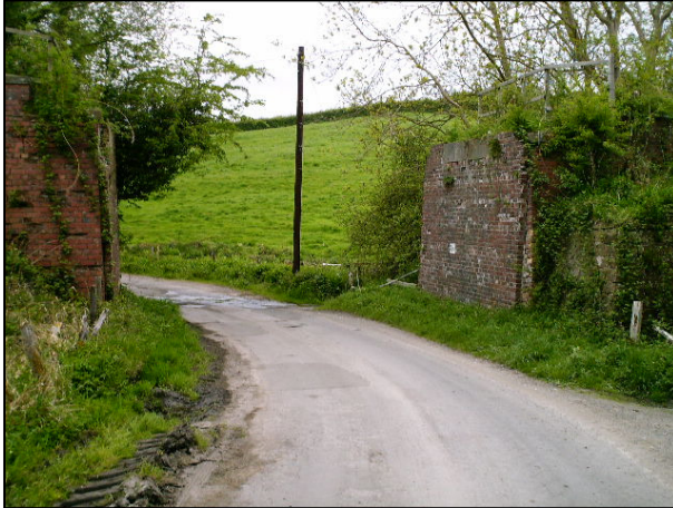
Abutments Prior to the works
