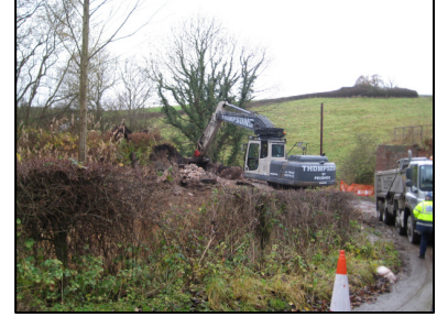
Demolition in progress
