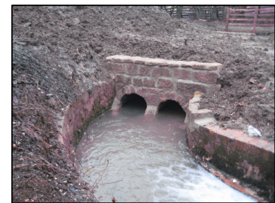
New Culvert Headwall
