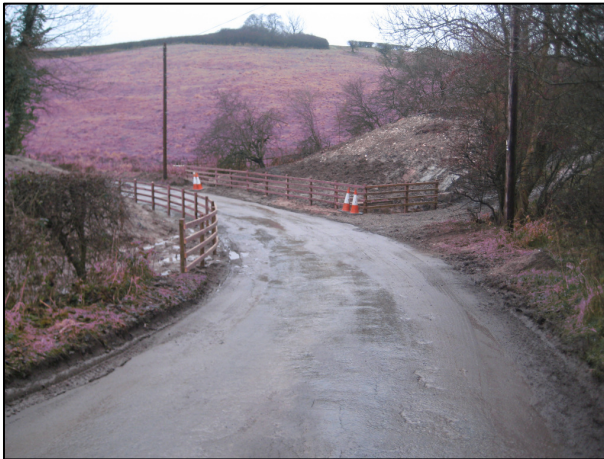
Works completed with landscaping and fencing
