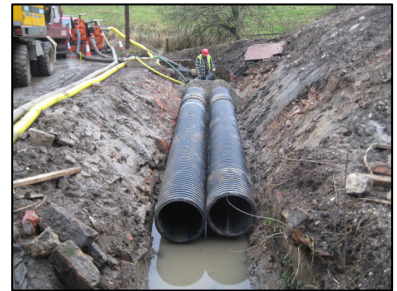
Culvert Construction in progress
