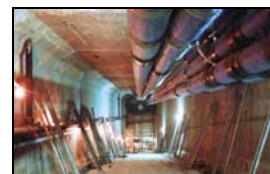
Additional tendons installed inside the box section
