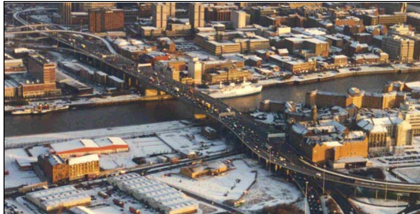
Kingston Bridge is a pair of bridges taking the M8 over the River Clyde
