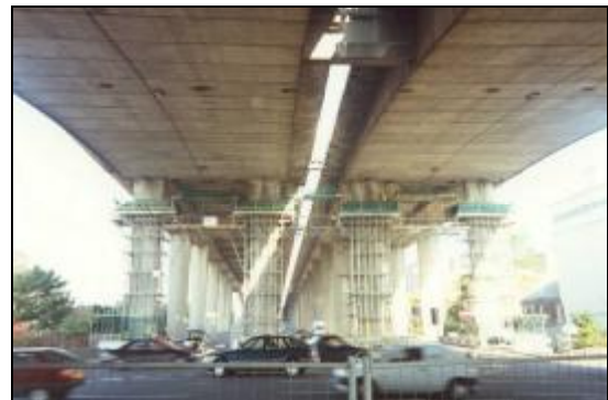
Temporary tie downs at the cantilevered end spans
