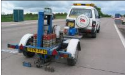
Each joint position was FWD tested
