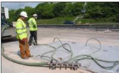
Applying the vacuum
