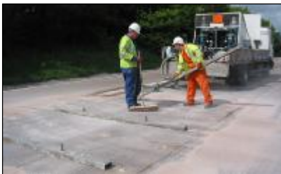
Preparing the treatment area
