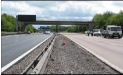
New inlaid blacktop and old concrete slab
