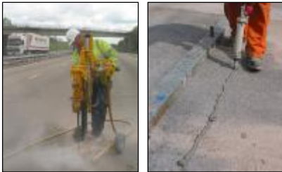
Drilling and sealant operations
