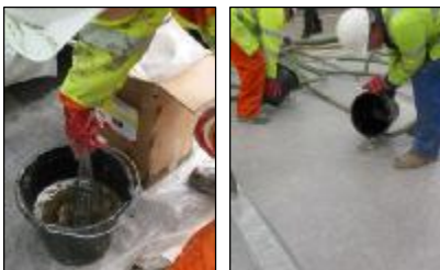
Mixing and introducing polyester resin
