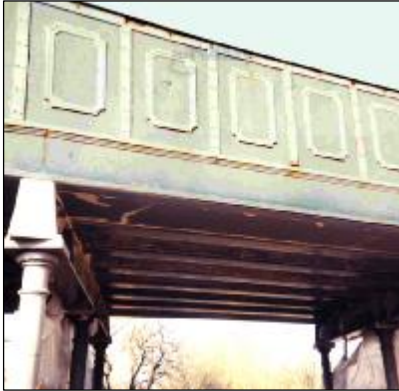
The bridge carries road over rail
