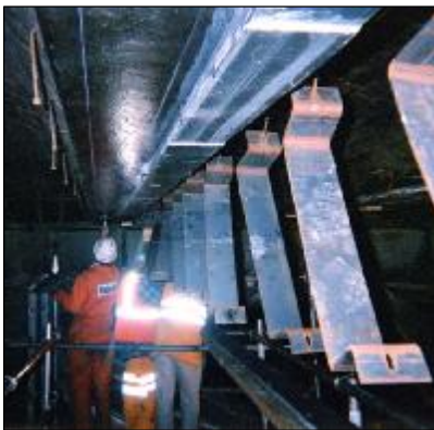
Preparing the cast iron beam
