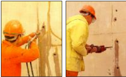
Resin injection can be highly effective
