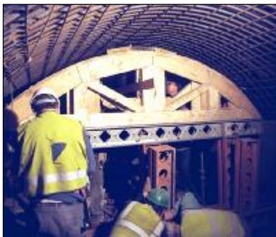
The arches were lined with RC concrete
