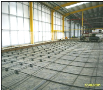
Conventional rebar reduced
