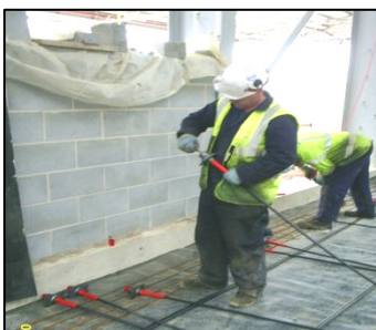
Dead anchorage installation
