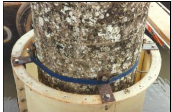
Temporary restraint of the FRP shuttering
