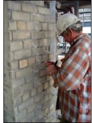
Ribbon anode installation in brickwork
