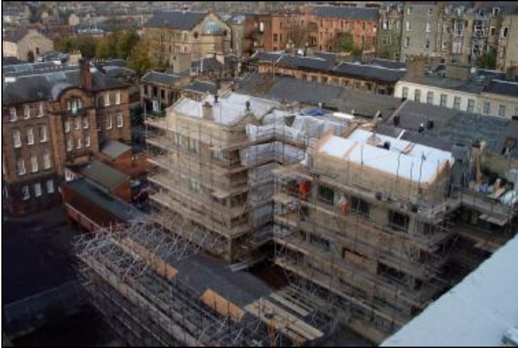
Complex scaffolding is required to access the structure
