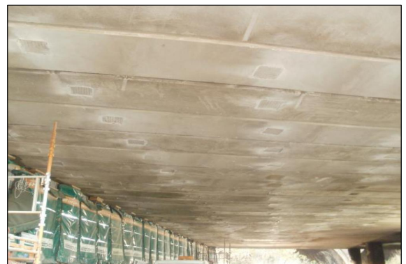
Repair of temporary prop locations following extensive spray concrete replacement and after shot of completed repairs
