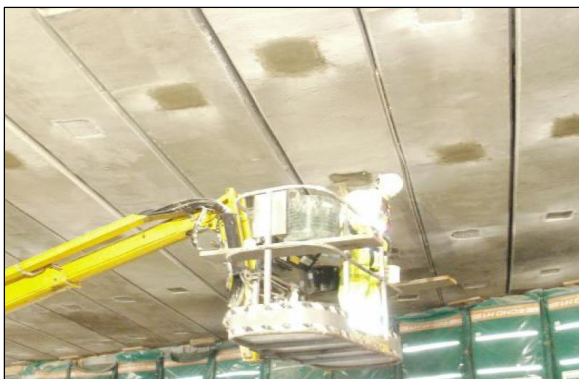
Repair of temporary prop locations following extensive spray concrete replacement and after shot of completed repairs
