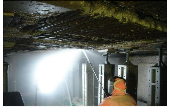
Hydro-Demolition of damaged concrete
