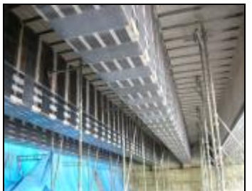
Scaffolding erected under the bridge
