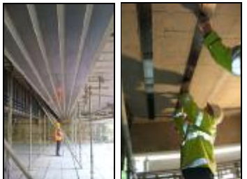
CFRP Plates bonded to the soffit
