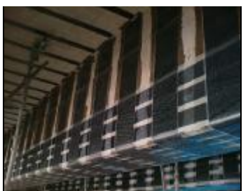
Carbon Fibre wrap was used to add extra strength
