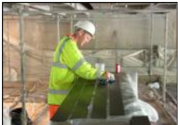
Preparing the CFRP Plates
