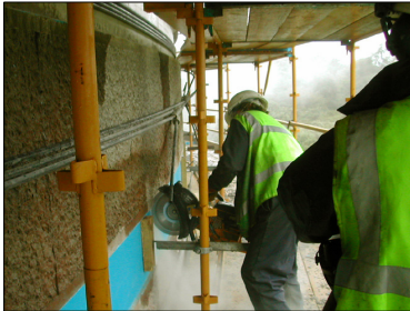
Strand cutting was carefully controlled
