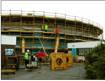
Four tanks were renewed at the Conlig site
