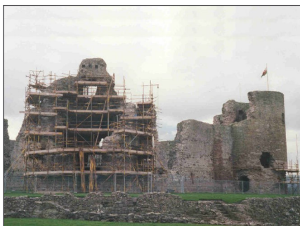
Heritage Structures - Restoration
