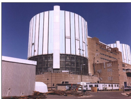
Industrial Premises - Repair
