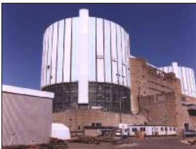
Industrial Premises - Repair
