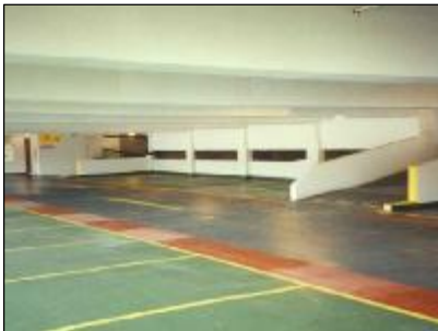
Car Parks - Renovation
