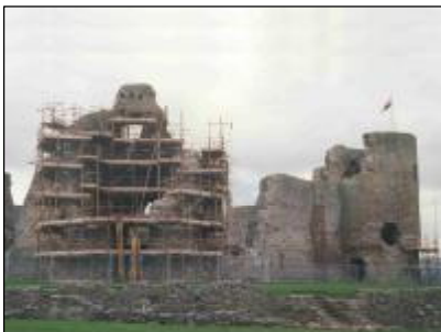
Heritage Structures - Restoration
