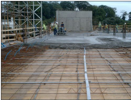
Conventional reinforcement is sparse
