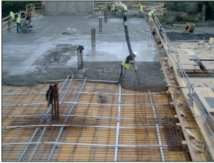
A floor slab being cast
