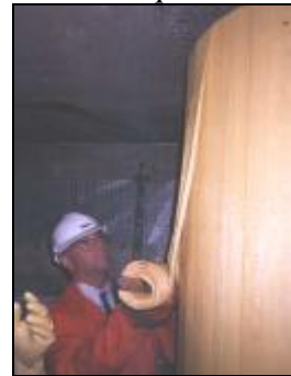
Kevlar® application to columns
