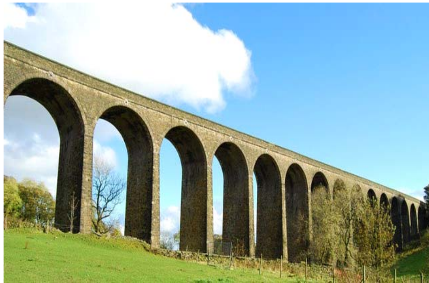
Above: Thornton Viaduct is a Grade II Listed structure
