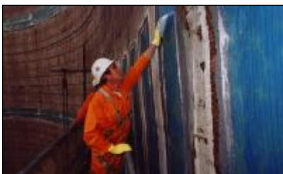
Applying the Kevlar ® fabric
