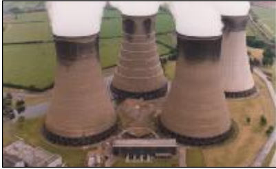
Cooling tower C1 (middle back)
