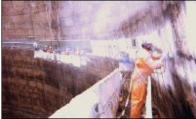
Preparing the concrete surface
