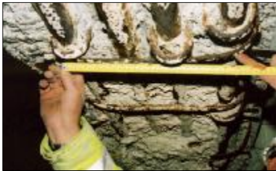
Hennebique designed beam reinforcement
