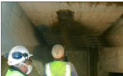
Repairs were made with sprayed concrete
