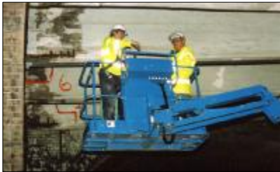
Access platforms were used frequently
