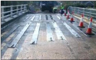
Steel plate bonding on the deck
