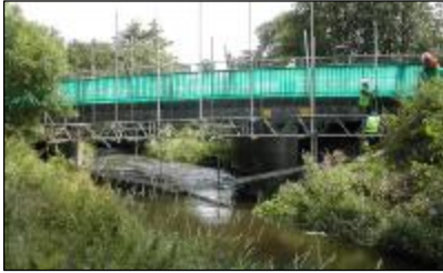
The bridge carries road over river
