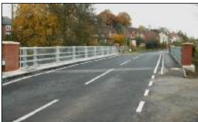
Re-surfacing to deck and approaches
