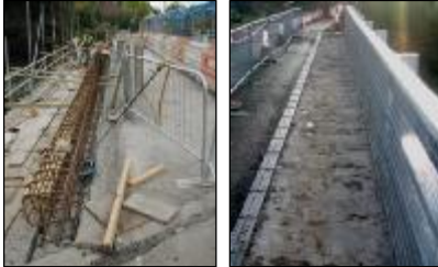
New stringcourses and parapets were built
