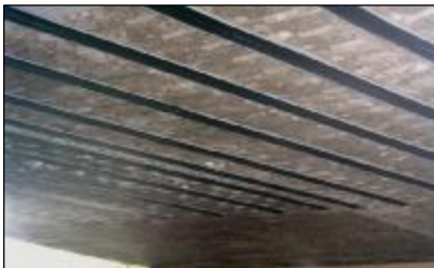
Carbon fibre plate bonding on the soffit
