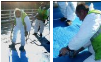
Spray waterproofing
