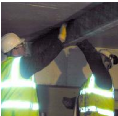
In all 700 beams were installed
