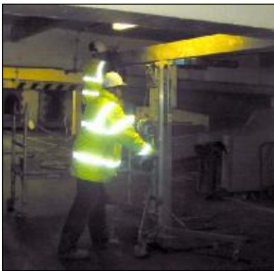
Installing a steel strengthening beam
