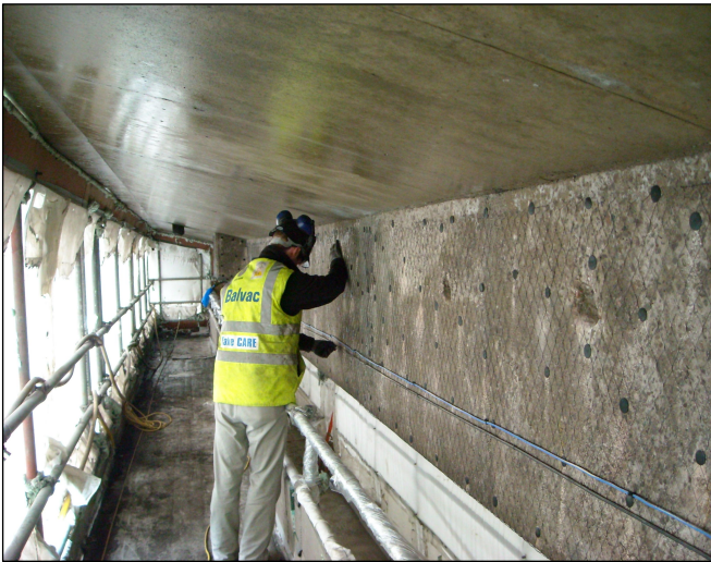
Operative Checking Mesh and Cable Installation
