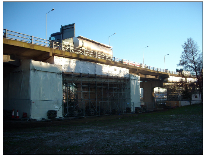
Widnes Approach Viaduct
