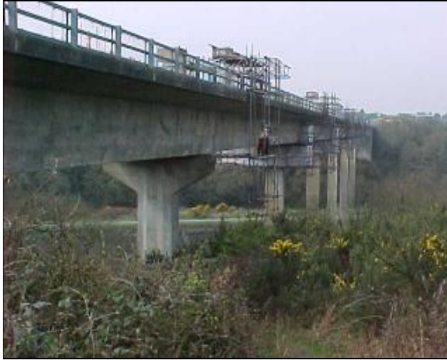
Westfield Pill Bridge carries the A477 over the Milford Haven basin
