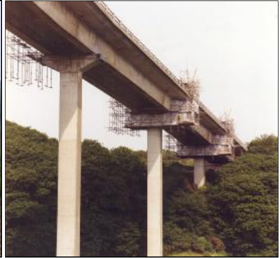
Suspended scaffolding provided access to the cross heads
