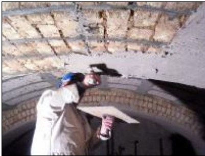
Lime plaster was chosen for authenticity
