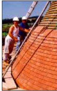
The roofs were strengthened and re-tiled
