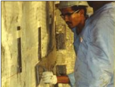
CFRP application to tower surfaces
