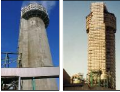
Prill tower: before and with access scaffold
