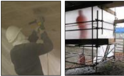
Edge cutting (L), hydrodemolition (R)
