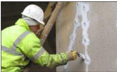
Preparing a crack for resin injection
