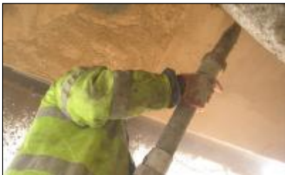
Sprayed concrete to soffit
