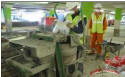
Mixing of repair mortar
