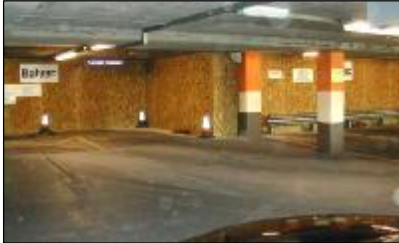
Traffic was protected from repair activity
