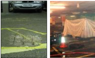
Spalling was removed by hydro-demolition
