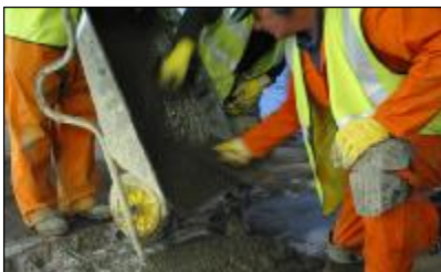
Placing of repair mortar
