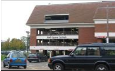
The car park remained open during repair
