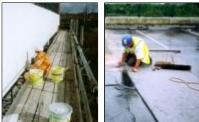
New coatings and mastic asphalt repairs
