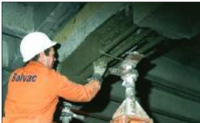
Concrete repairs required temporary works
