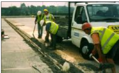
ACO drains were replaced .....
