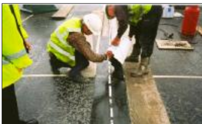
..... and expansion joints renewed
