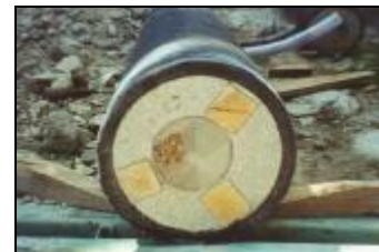
Coloured grout shows the filled void
