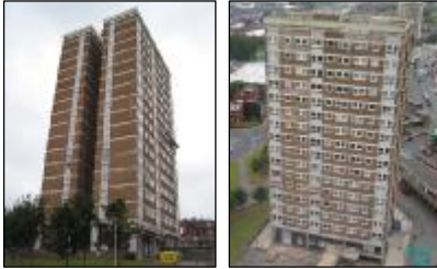
Two of the four tower blocks
