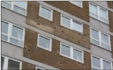
Repointing and brick replacement
