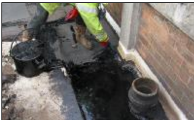
Re-roofing with high spec mastic asphalt
