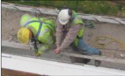
Most work was carried out from cradles
