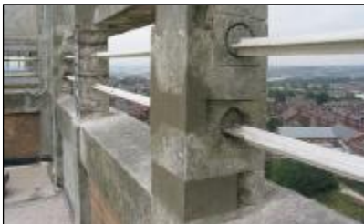
Concrete repair to roof parapets
