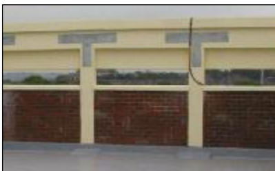
Steel plate strengthening of parapet
