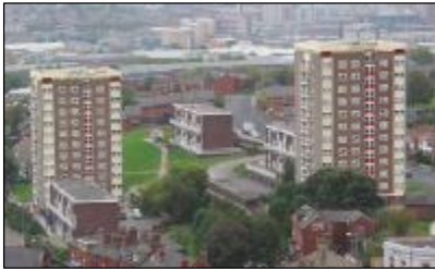
Two of the four tower blocks in Armley
