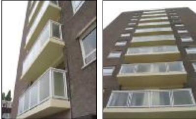
Repairs to balconies and brickwork
