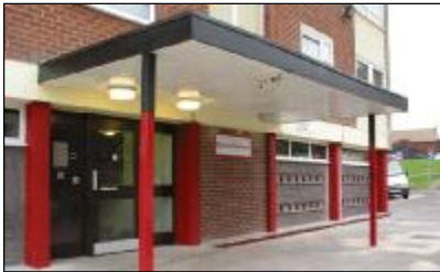
Refurbished entrance canopy
