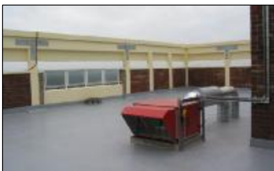
New roofing and extraction plant
