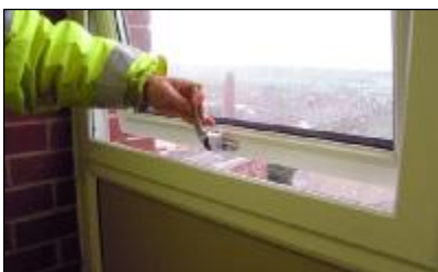
Replacement UPVC windows
