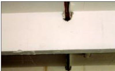
..... and the lighting replaced and upgraded
