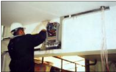
Cathodic protection was installed .....
