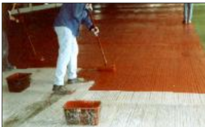
All decks were waterproofed .....
