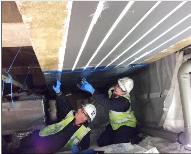
Application of CFRP Wrap over bonded CFRP Plate
