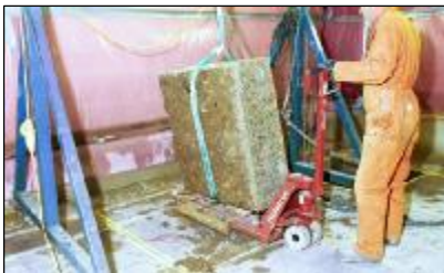
Controlled lifting of slab sections
