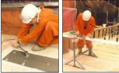
Steel plate bonding
