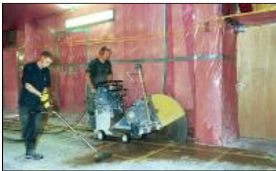
Saw cutting of floor slab into sections
