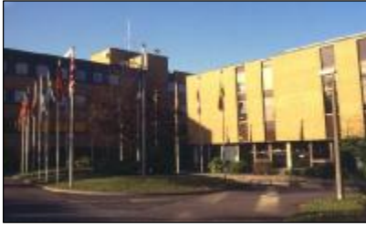
European Weather Centre Building
