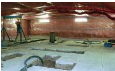
Removed slab sections within enclosure
