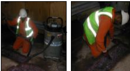
Waterproofing and concrete repair
