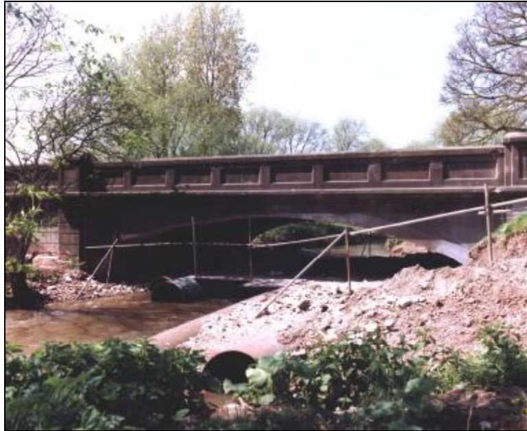
Washford Bridge required a complete refurbishment and strengthening
